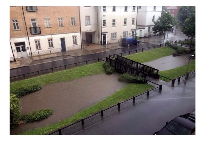
A great example of Sustainable Urban Drainage Systems (SuDS) working successfully was on our residential service charge site at Upton in May 2018, when heavy rainfall in Northampton caused flash flooding in the area.
